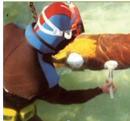
Figs. 1a and 1b: Examples of high performance coating (a) glass flake reinforced polyester coating to achieve 1000µm in one coat (b) underwater coating on the tidal zone
